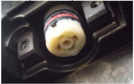
3. Use the same Allen key/wrench to remove the valve-insert the key into the center of the valve
